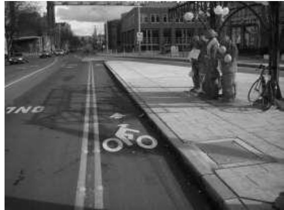
Figure 17: Contraflow Bike Lane Photo Source: Seattle Department of Transportation
