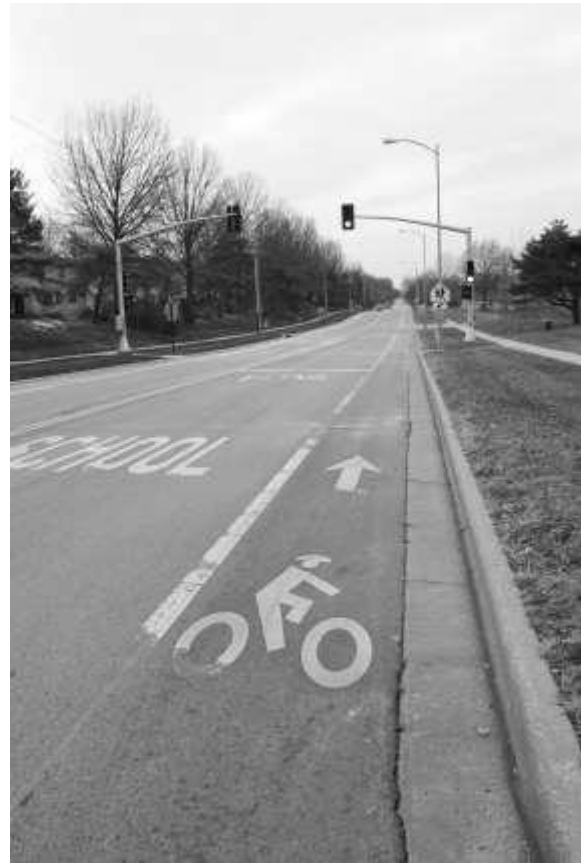
Figure 5: Bicycle Lane Photo
