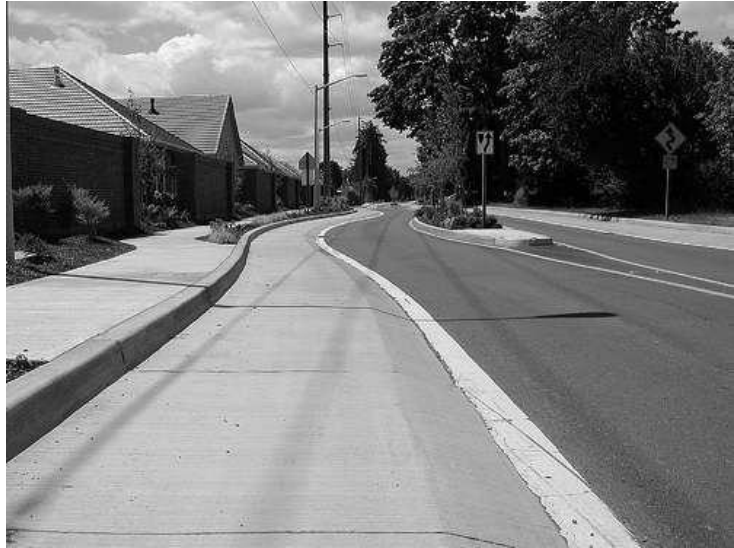
Figure 20: Raised Bicycle Lane Photo
