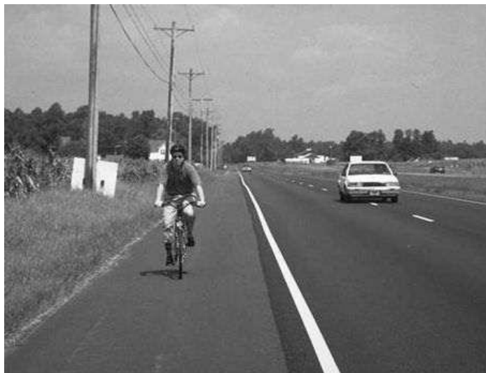
Figure 2: Paved Shoulders Photo
