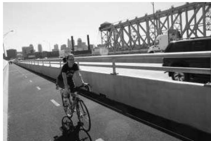
Figure 36: Sidepath Along Bridge Photo
