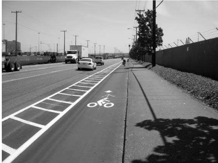
Figure 19: Buffered Bicycle Lane Photo
