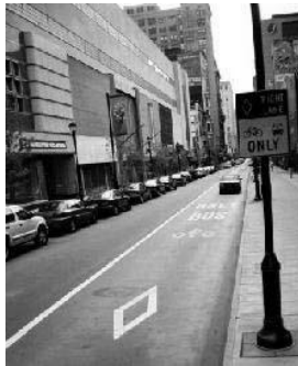
Figure 31. Bus/Bike lane, City of Philadelphia, PA.
