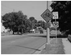
City of Olathe, KS North Gate Road Asphalt Wide Curb Lane 13 foot with cautionary “Share the Road” sign.
