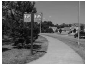
City of Shawnee, KS Blackfish Parkway Trail Class I Multi Use Path 10 foot.
