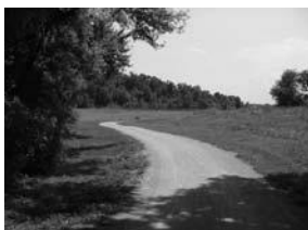
Jackson County, MO Little Blue Trace Trail Crushed Limestone Class I Multi Use Path 8 foot.
