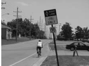
City of Olathe, KS Dennis Ave. Asphalt Bike Lane 4 foot.
