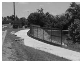
City of Kansas City, MO Indian Creek Trail Concrete Class I Multi Use Path 10 foot with center strip.
