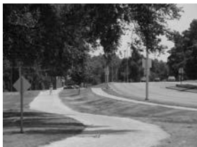
City of Kansas City, MO Trolley Track Trail Crushed Limestone Class I Multi Use Path 8 foot.
