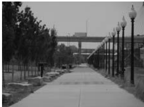
City of Kansas City, MO River Heritage Trail Concrete Class I Multi Use Path 12 foot.
