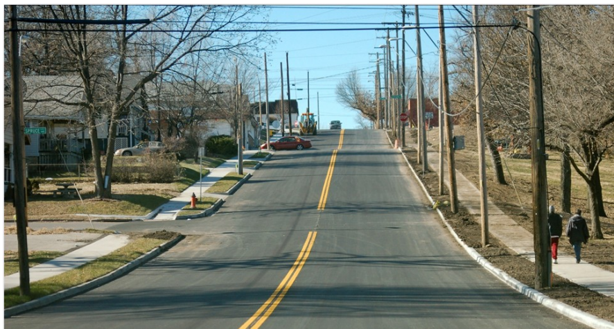
39 th Street (Cleveland to Elmwood) After
