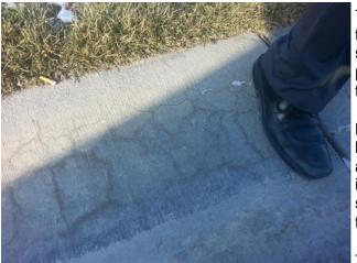
Todd LaTorella of the <u>American Concrete Paving Association</u> met me at the subdivision to examine the curb. Curb throughout the subdivision had surface cracking similar to D-cracking (see the photo), but because it had pink quartzite coarse aggregate, we knew that it wasn't D-cracking and thought perhaps that low air entrainment was the culprit.
