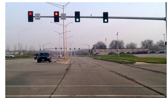
By communicating with each other, the traffic signals can intelligently adapt to traffic demand. In this picture, you see several intersections turning green at the same time.
