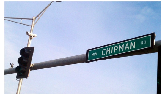
A mast arm on Chipman Rd. with mounted IP video camera for vehicle detection.
