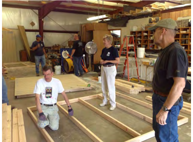
David Brackey, Lois Belser and Dennis Bar work on framing.
