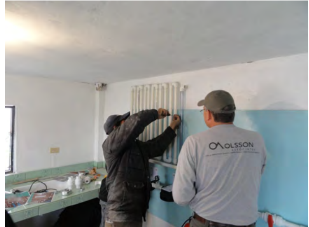
Installation of a system.
