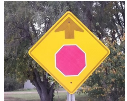
Right picture: Black border and arrow fading in less than 5 years
