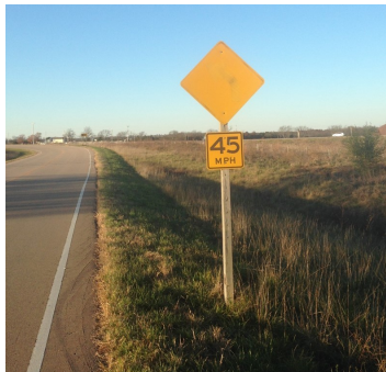
Left picture: Curve sign less than 5 years old installed on KDOT project
